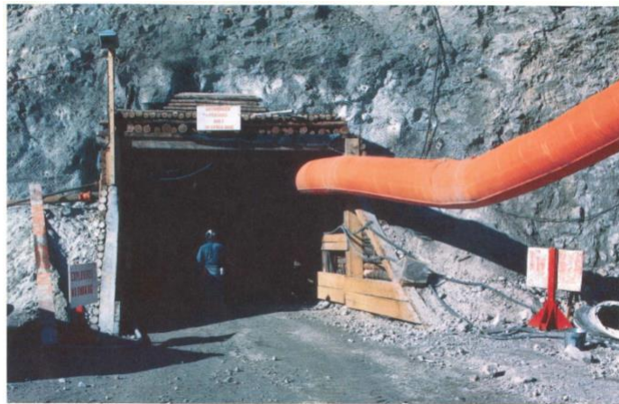
The underground mine project started in 1984; above, the portal in the pit wall.
